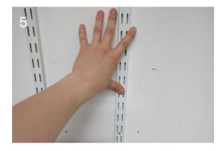
Take care that when joining rails vertically, that the distance between the top and bottom slots of new rails are equal to that of all slots on the rails.
