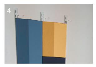
Insert panel hooks into rail slots then push down to slide into place. Always ensure that panels are installed starting at the bottom and working up.
