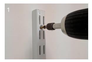
Fix bottom left or right rail onto wall, starting with the top screw hole.
