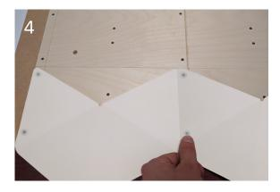
Select the next main tile. Place this tile into position, ensuring that the holes on the left of this tile align with the open holes on the tile to the immediate left and use the mounting pegs to attach these together.
