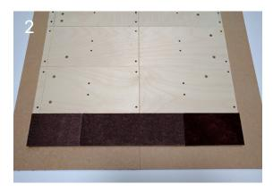
Once the bottom row is complete, continue adding main mounting boards above, ensuring all boards are aligned.
